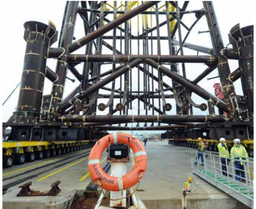
Transport of a jacket for an offshore substation weighing 1,850 t with 2x 30 axles
