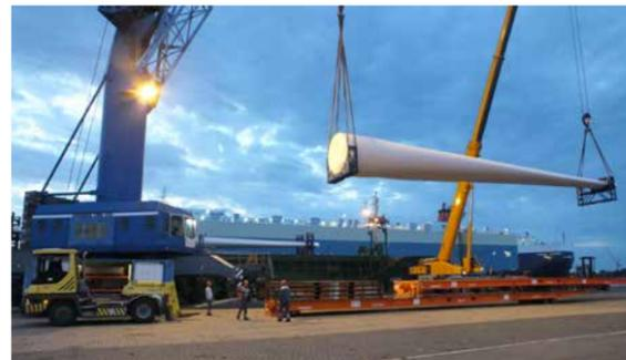
Twin lift crane operation ex/on barge or coaster.
